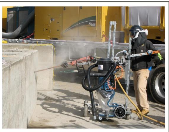
Drilling with the jig, no vacuum
