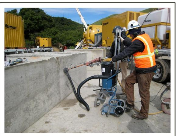
Drilling with the jig and vacuum
